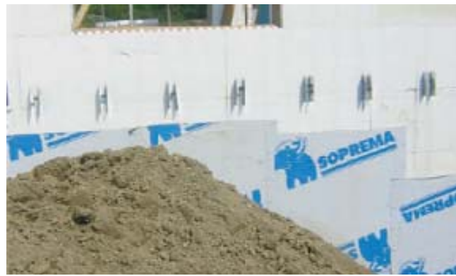
Peel and stick membrane installed and ready to be backfilled
