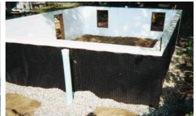
Installed dimple sheet membrane
