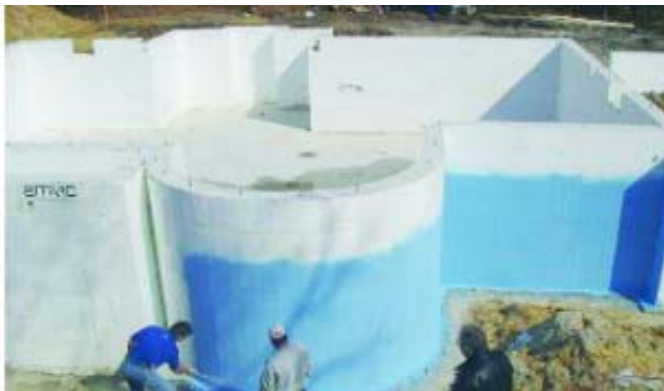
Spraying liquid applied membrane
